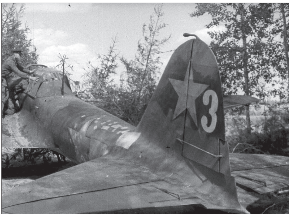
Il-2 s/n 1863514, tactical number 3, from the 61st ShAP, August 1941. The airplane was painted in improvised black-and-green camouflage of the Factory No.18, with enlarged insignia applied in six positions.
