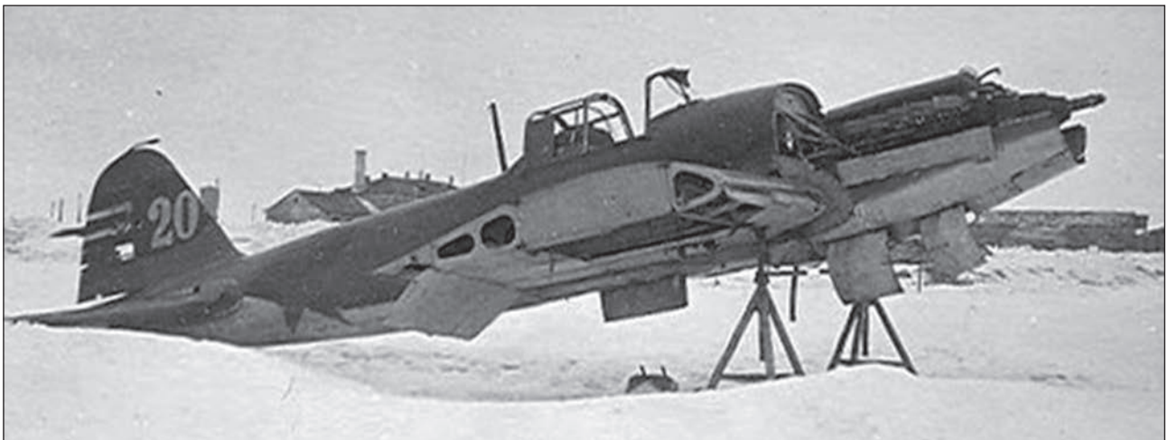
Il-2, tactical number 20, of an unknown unit, captured by the enemy at an airfield, autumn 1941. The airplane was painted in improvised black-and-green camouflage of the Factory No.18, with enlarged insignia applied in six positions.
