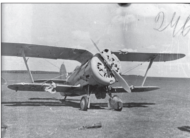
I-153 s/n 8030, tactical number 6, of the 160th IAP. This was one of the last aircraft manufactured by Factory No.1, and was painted according to the earlier scheme, using AI light grey aircraft lacquer.
