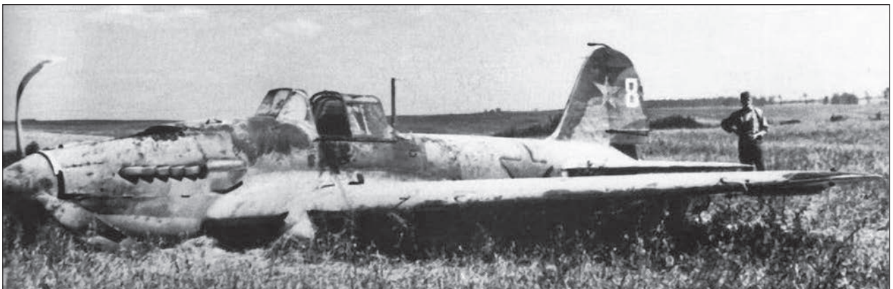
Il-2, tactical number 8, of an unknown unit, captured by the enemy at the airfield, August–September 1941. The airplane was painted in improvised black-and-green camouflage, with insignia in six positions – four of increased size and the stars on the tail fin of the earlier (smaller) size.
