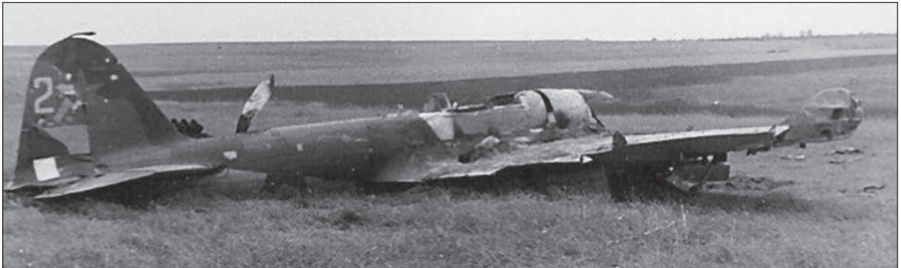
Il-2, tactical number 2, of an unknown unit, captured by the enemy at the place of forced landing, August–September 1941. The airplane was painted in improvised black-and-green camouflage, with insignia in six positions – four of increased size and the stars on the tail fin of the earlier (smaller) size.
