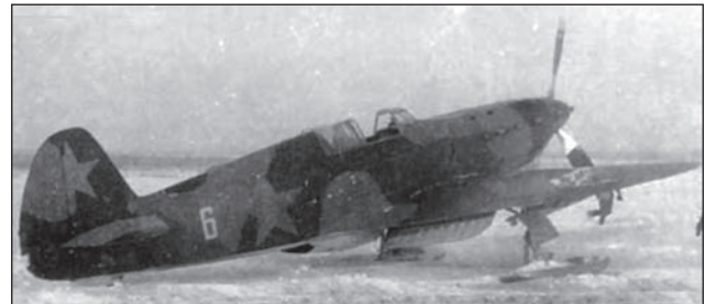
Yak-1 of the 43rd–44th series, tactical number 6, captured by the enemy at the place of forced landing, winter 1941–1942. The airplane was painted in black-and-green camouflage, according to the scheme attached to the SNK Directive No.1711, with enlarged insignia applied in six positions.
