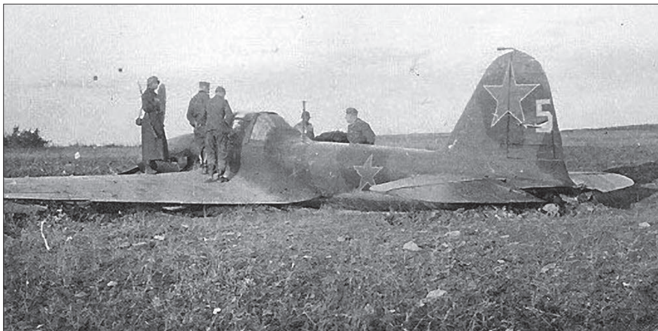
Il-2, tactical number 5, of an unknown unit. The airplane was painted in improvised black-and-green camouflage, the insignia with white edging applied in six positions, and a star of reduced size on the fuselage.
